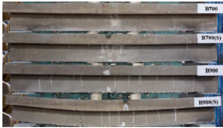
Fig. 6—Visible damage of RC T-beams after exposure to fire.
